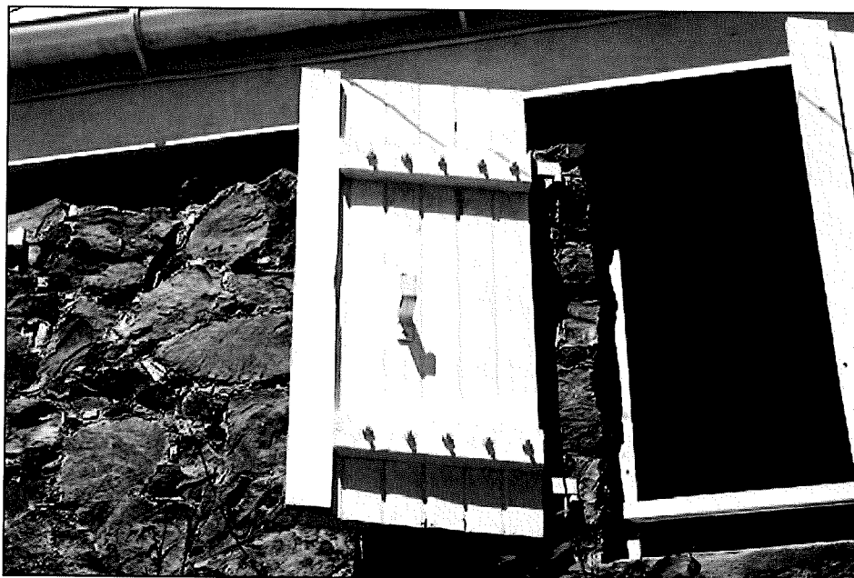
Figure 11-9. Very old building with robust shutters constructed of 2x4 lumber, bolted connections, and heavy metal hinges. Hurricane Marilyn (U.S. Virgin Islands, 1995)
