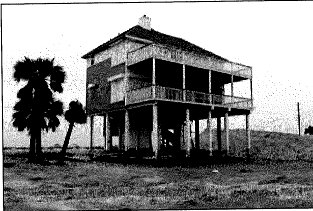
Figure 10-8. Scour around grade beam, Hurricane Ike (Galveston Island, TX, 2008)
