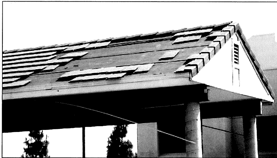
Figure 11-50. Tiles that were nailed to thin wood sheathing. Northridge Earthquake (California, 1994)
