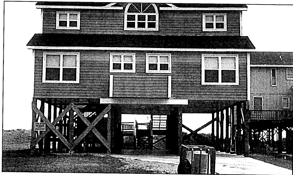
Figure 10-10. Diagonal bracing using dimensional lumber
