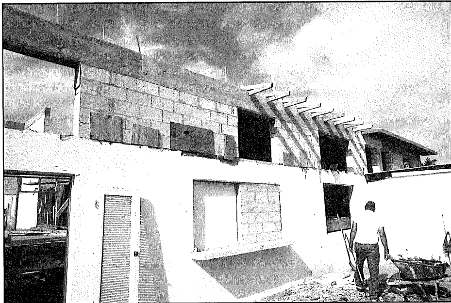
Figure 67 The extended first- story walls.
